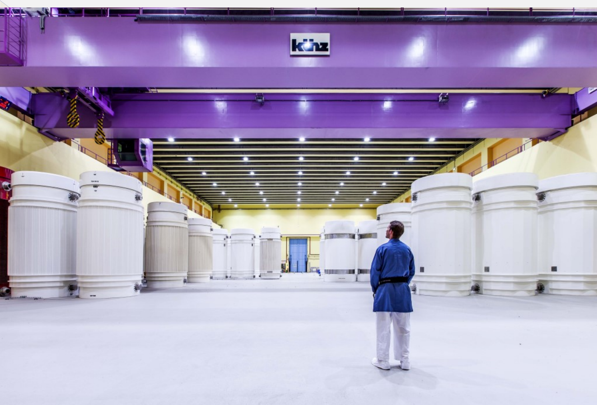
Interim storage facility ZWILAG for HLW and LLW/ILW
